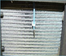
Electronic or Thermistor probe attached to evaporator coil
